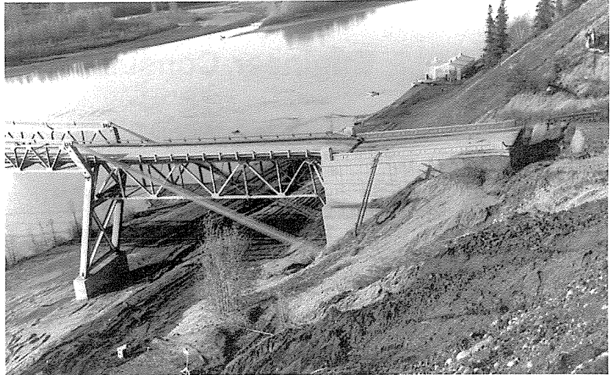
Fig. 2. Collapse of Peace River highway bridge at Taylor B.C. on 16 October 1957. Courtesy University of Alberta Archives
