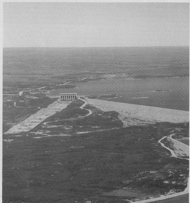
James Bay Complex. LG - 2. Main dam and spillway. (Photo credit: Hydro-Québec).
