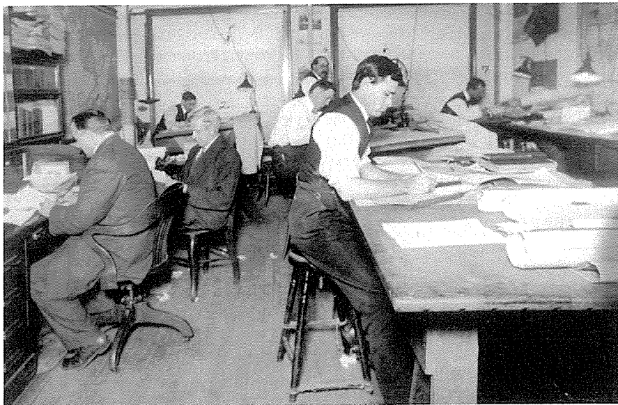
1. Grand Trunk Pacific bridge design office. O. K. Peck in right foreground. J. G. Legrand at desk to left.
