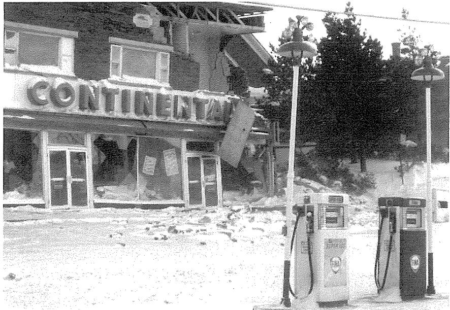
Fig. 2. The failure extended into the town. The damage to this store was extensive. Fortunately there were no casualties.
