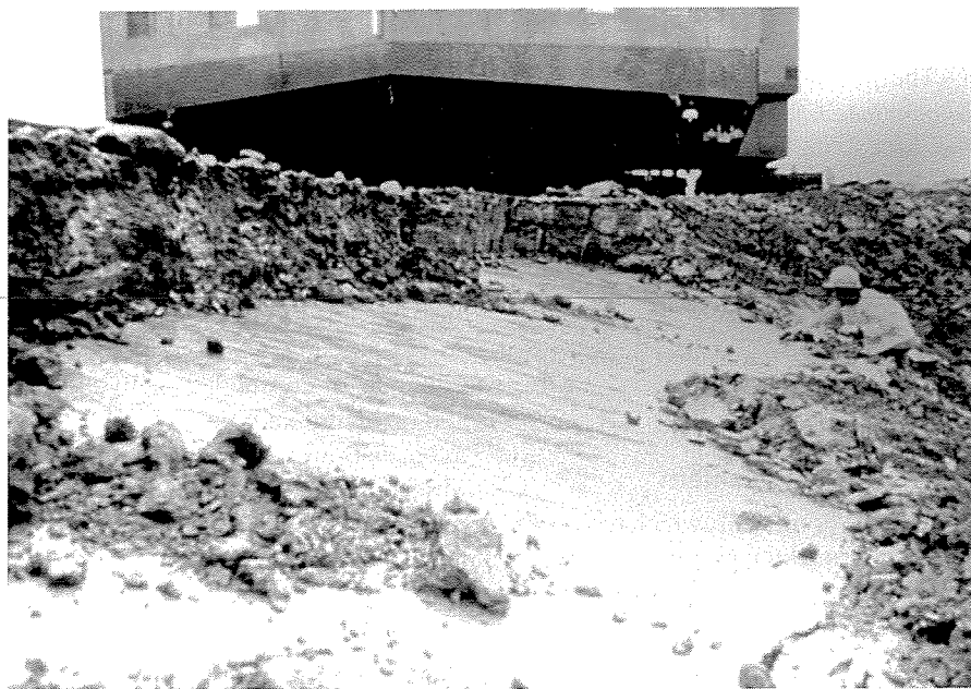
Fig. 4. Shear surface on dipping clay bed; dragline in background.
