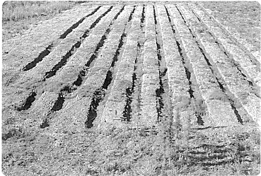
Trials of ditching in permafrost for buried pipelines backfilled with excavated spoil which subsequently thawed out.
