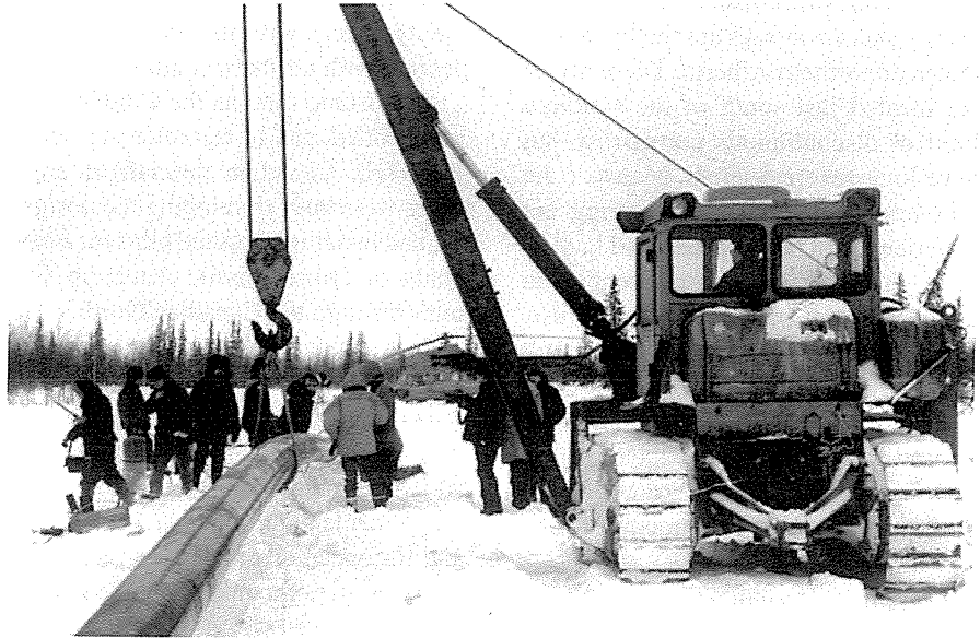
Russian side boom lifting pipeline on total project. [Photo Credit: Al Hanna]
