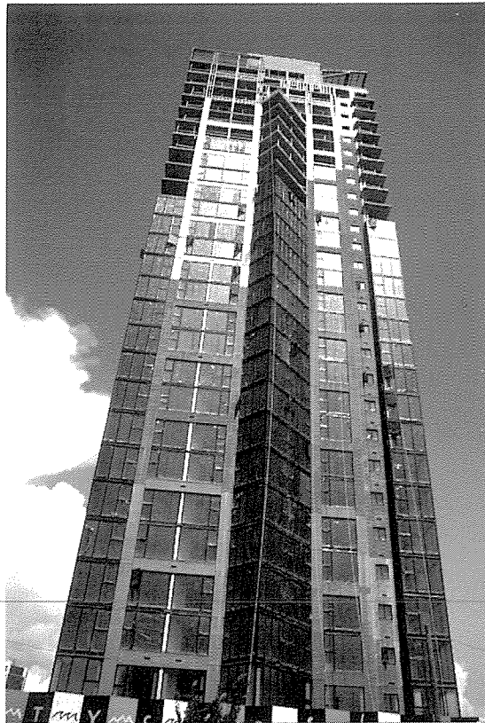
Fig. 6. City Crest Tower, Vancouver, B.C.
