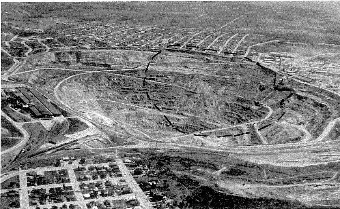
Fig. 1. Canadian Johns Manville pit at Asbestos, Quebec. The slope adjacent to the town failed due to the sudden infiltration of water from a broken high-pressure water main. Over 30 million cu. yds. of material was involved. The slope was stabilized by a combination of unloading, horizontal drain installation and drainage into an underground adit.
