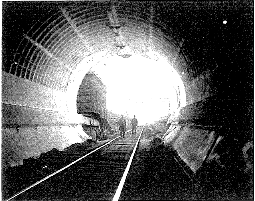
Photo 6. St. Clair Tunnel, Interior View 1908, National Archives.
