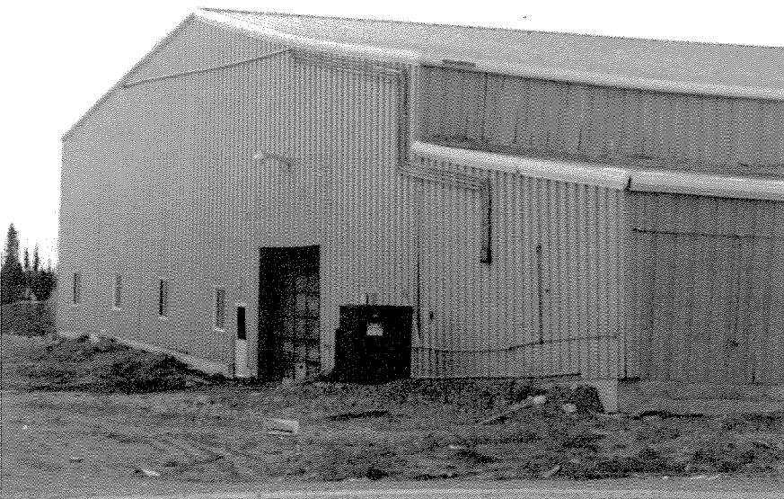
Rear of aircraft hanger built in discontinuous permafrost zone with differential thaw settlement visible along window line.
