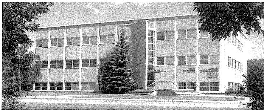
Photo 8. The PFRA Soil Mechanics Building, later renamed the Robert Peterson Building, on the University of Saskatchewan Campus.
