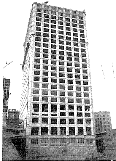
Fig. 8. Nearly completed Oxford Tower, (McCauley Plaza), Edmonton, 25 October 1968.
