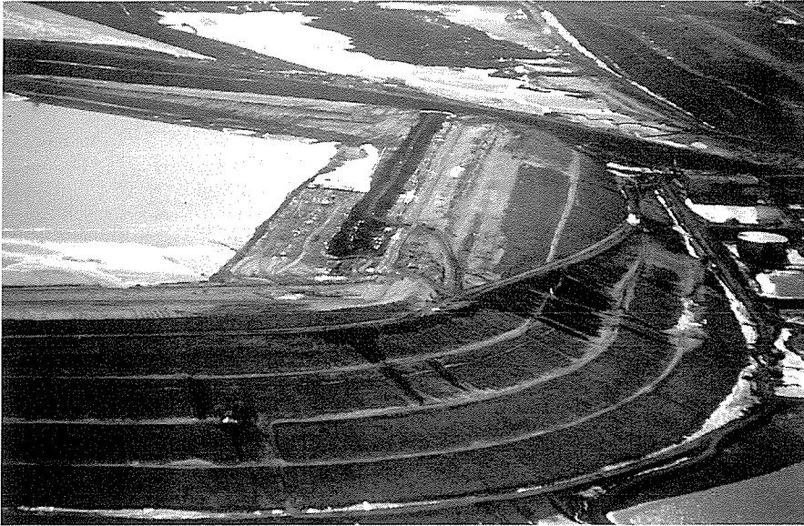
Fig. 5. Tar Island Dyke - north-east corner of tailings pond constructed mainly of hydraulically placed sand, 8 April 1976. MCH Photo
