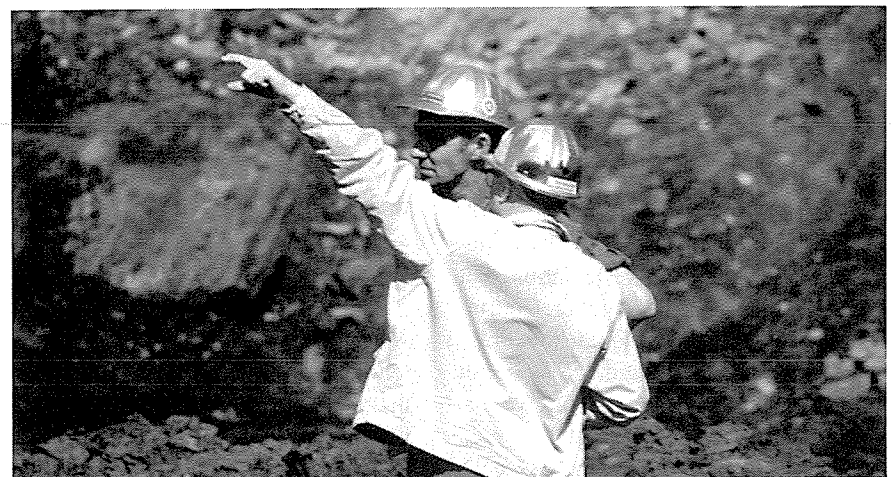
Fig. 4. "This is what happens, Scotty", Shell Test Pit in oil sand, 4 July 1975. MCH Photo
