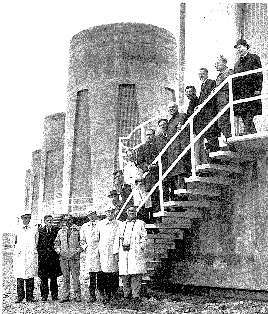
Photo 10. Robert Peterson with PFRA officials and visiting geotechnical engineers at the Gardiner Dam control towers.
