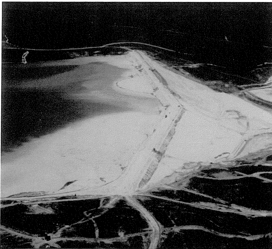
Fig. 10. Aerial view of L-L Tailings Dam Highland Valley Copper Mine.
