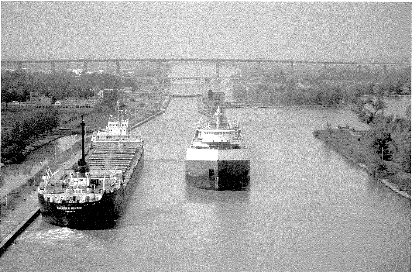
Welland Canal (Courtesy of The St. Lawrence Seaway Authority).
