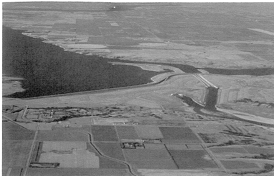
Photo 2. View of Gardiner Dam and Lake Diefenbaker in central Saskatchewan.
