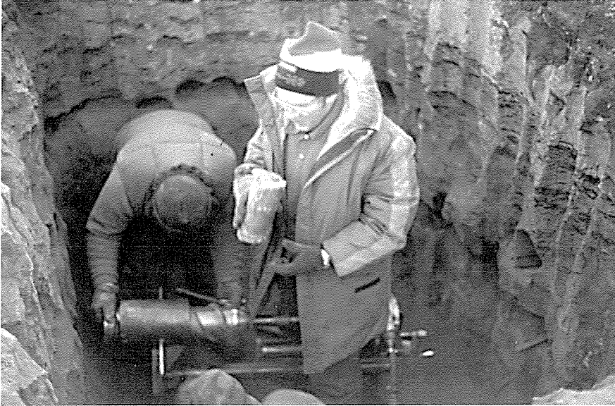
Horizontal coring program to obtain undisturbed samples of ice rich soil for studies of lateral loading interactions of creep in buried pipelines.
