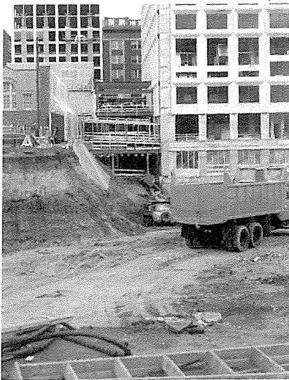
Fig. 7. Excavation for Oxford Tower, (McCauley Plaza), Edmonton, 17 October 1968.
