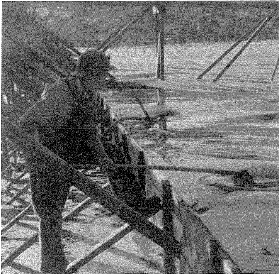
Fig. 4. Upstream dam construction, B.C. (Early 1950).
