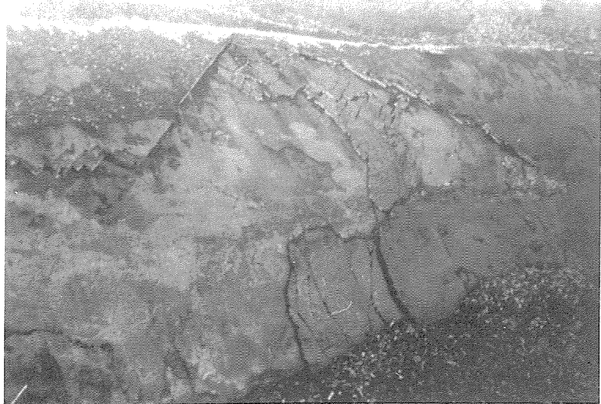
Fig. 5. A major buckling failure which occurred at the Line Creek Mine, B.C. in thinly layered bedded shale underlying the lowest coal seam. After removing the unstable slab, pattern bolting and pattern horizontal drains were installed to develop stability.
