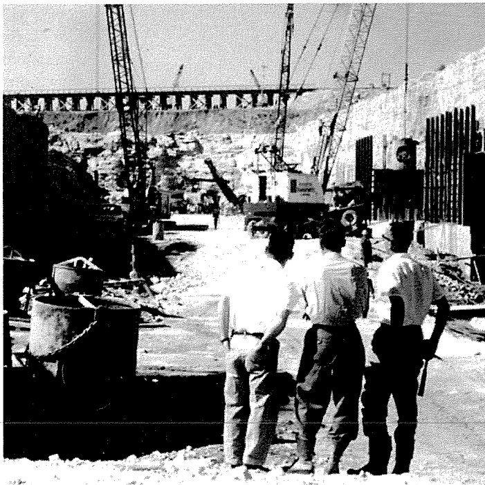
Fig. 2. Starting construction of lower Beauharnois lock. Railway trestle in background to be diverted, then bridged across lock gate.
