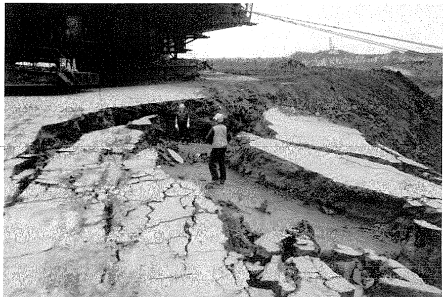
Fig. 6. A block slide that occurred at the crest of the highwall at Syncrude. Monitoring staff alerted the dragline operator who immediately began to move the machine away from the movement. Note the clay layer which dips toward the highway.
