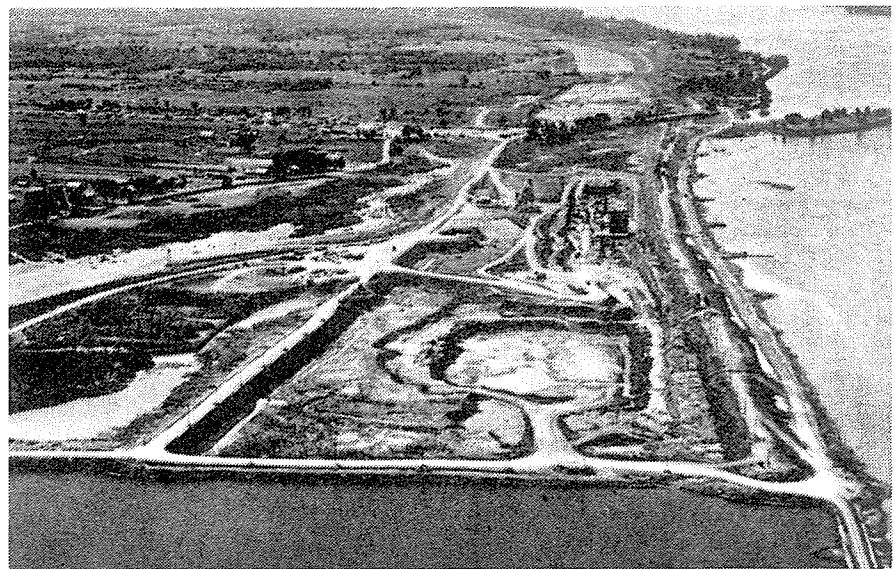
Fig. 4 Aerial view upstream from Côte Ste-Catherine with Lachine Rapids in the distance. Lock construction is starting within the cofferdam. Channel excavation extends in the distance.
