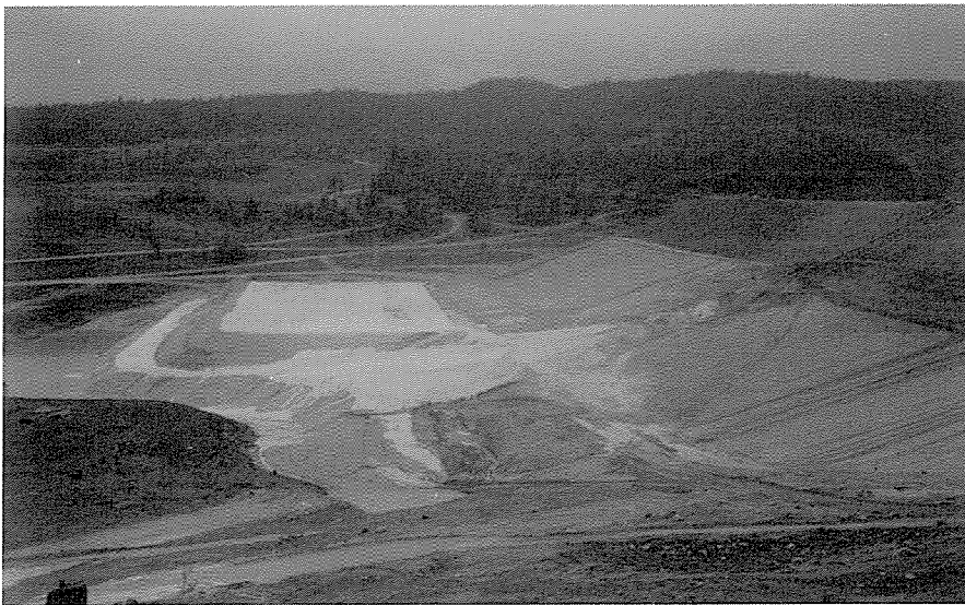
Fig. 9. Photo looking along downstream slope of L-L Tailings Dam, Highland Valley Copper Mine.
