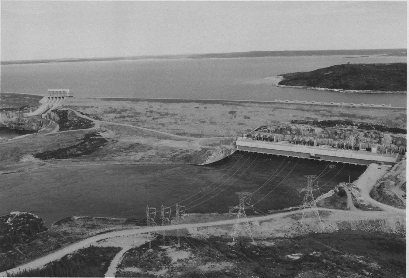
James Bay Complex. LG - 3. South dam (Main dam). (Photo credit: Hydro-Québec).
