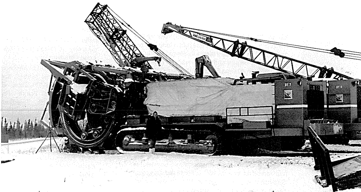
Arctic ditcher trials of equipment capable of excavating ditch in permafrost for large diameter buried transmission line. [Photo Credit: Al Hanna]
