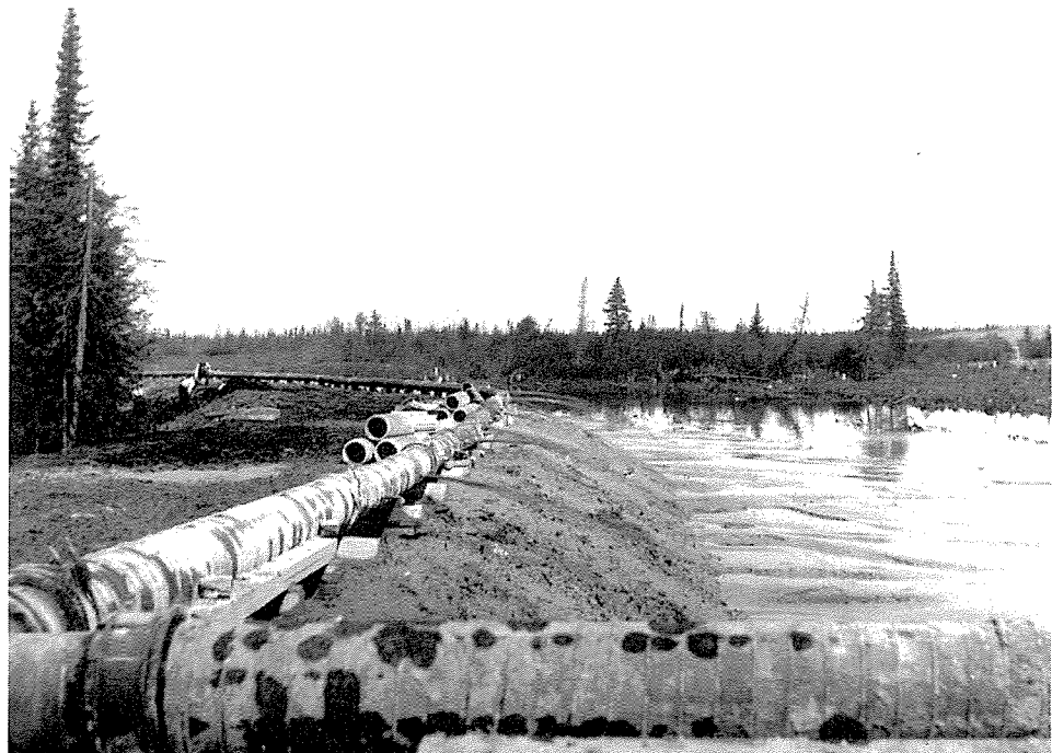
Fig. 3. Upstream dam construction, Hollinger Mine, Ontario (1936) (National Archives of Canada PA 017613).
